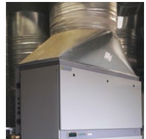
Example of duct installation
